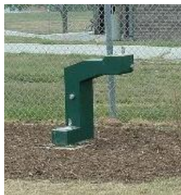
Water Fountains have been installed!
